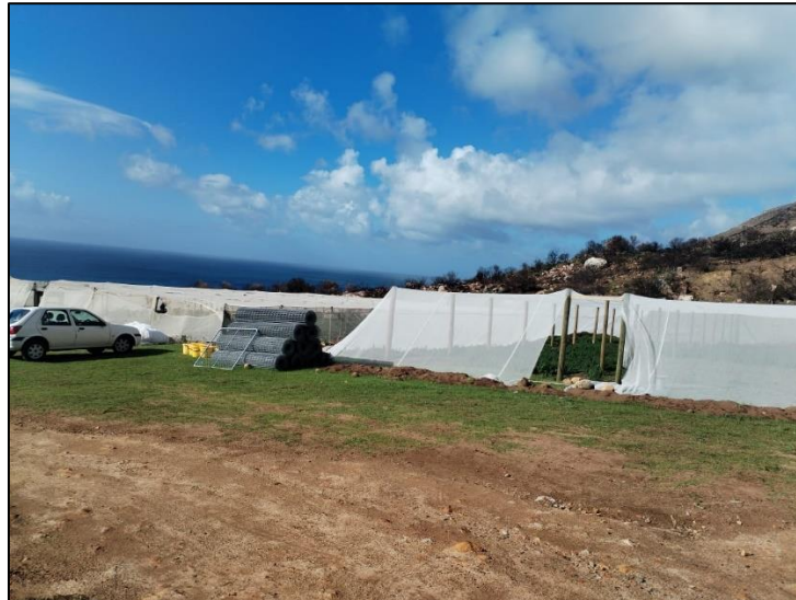
Figure 9. Vegetable tunnel repairs are underway at Rocklands Farm.
